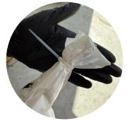
BUNCH UP ONE END LIKE SHOWN IN THE PICTURE AND PLACE CABLE TIE AROUND TUBE, TIGHTEN SECURELY.
